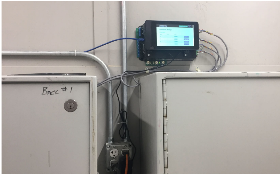
Fig 4 CHANGERVVIEW unit on site - connected to 2 Standard SC 34RL- DA machines, total 4 bill acceptors.
