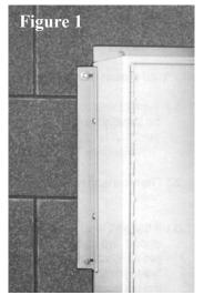
Some rear load models have the coin hoppers mounted on the door. When the hoppers are full and the door is opened, a significant load occurs on the cabinet. <u>This load can result in cabinet flexing if the cabinet is not sufficiently supported.</u> Repeated flexing of the cabinet can result in metal fatigue and stressed weld joints on the cabinet.
